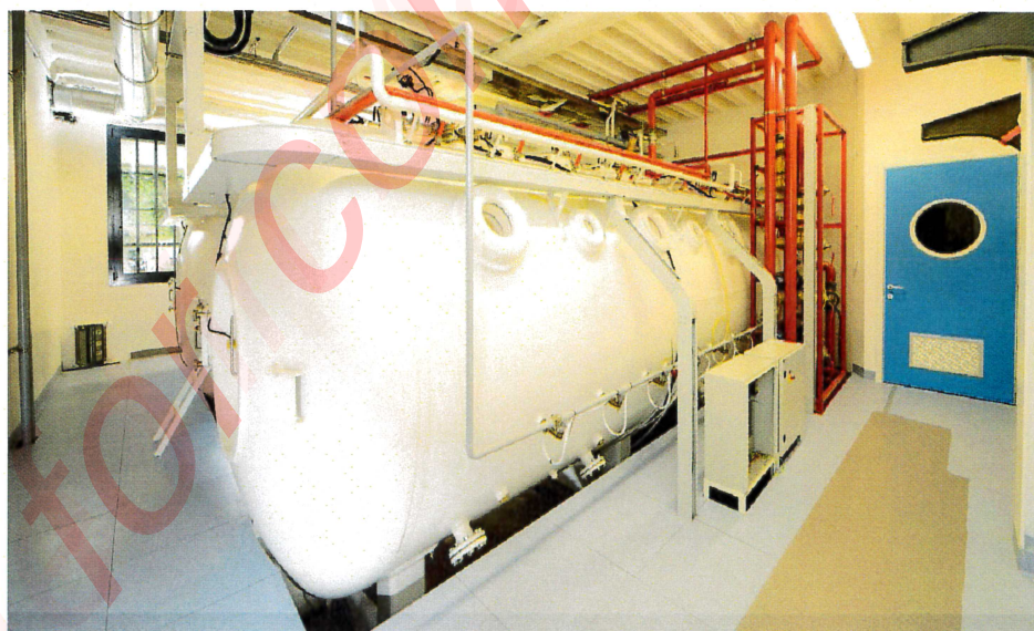
Figure 4. Rear view of the hyperbaric chamber. Sprinkler lines can be identified (red) and the portholes (on both walls) of larger size for direct vision inside the room and to admit light from outside. Smaller portholes are used to house video cameras to record activities inside the chamber.
