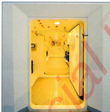
Figure 3. Main entry through the airlock which is made up of a rectangular door with an O-ring.
